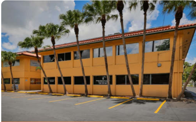
10250 Southwest 56th Street
