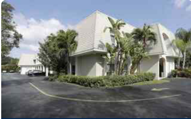
8353 Southwest 124th Street
