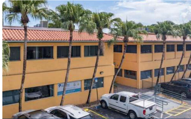
10250 Southwest 56th Street
