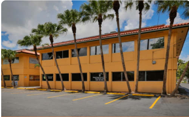
10250 Southwest 56th Street
