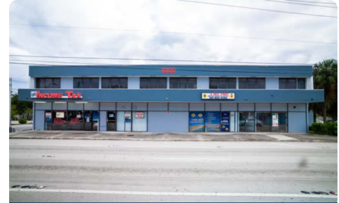
1000 E Atlantic Blvd, Pompano Beach
