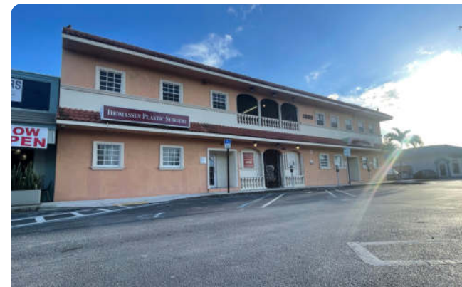
2800 E Commercial Blvd Fort Lauderdale, FL
