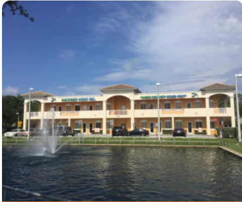
4100 Davie Road Extension, Hollywood, FL
