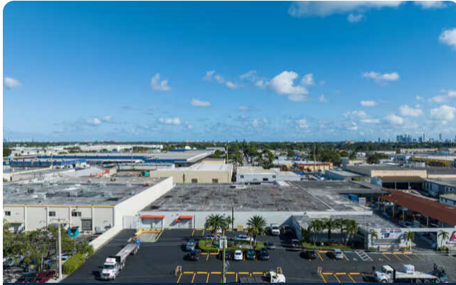
6865 Northwest 36th Avenue
