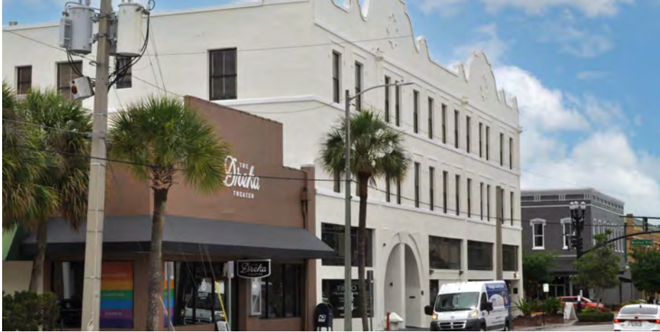
D 112 E New York Ave DeLand, FL 32724
