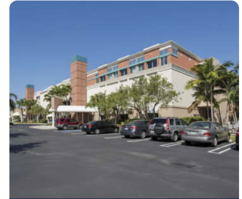
7785 Northwest 48th Street
