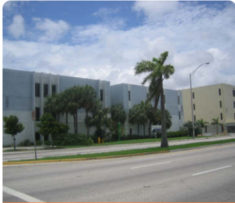
6595 Northwest 36th Street
