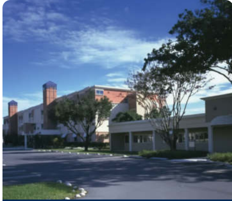
7705 Northwest 48th Street
