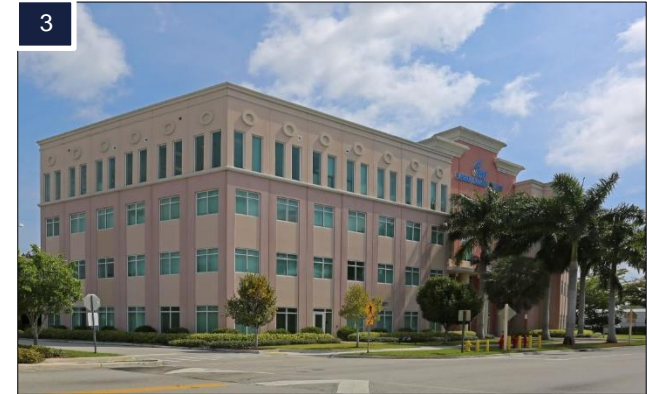
11731 MILLS DRIVE 11731 Mills Drive , Miami, FL, 33183
