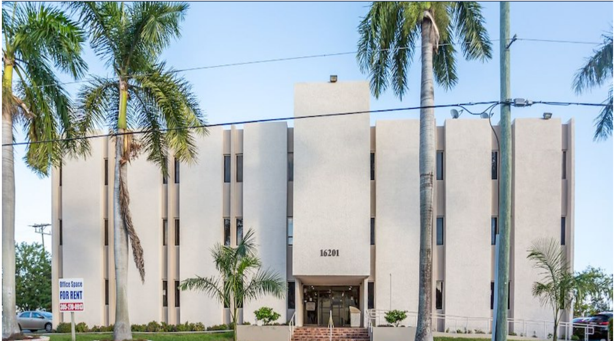
CHICAGO FINANCIAL BUILDING 16201 SW 95th Ave • Miami, FL 33157
